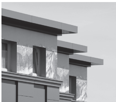
Long-term renewal and maintenance with cost-effective modernisation using ALUCOBOND®: Höxterstraße in Hagen, Germany
